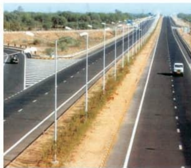
Fig. 7.2: Ahmedabad- Vadodara Expressway
